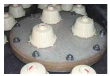
Internal Nozzle Plate Service Hatch
