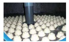
Nozzle Plate under drain system
