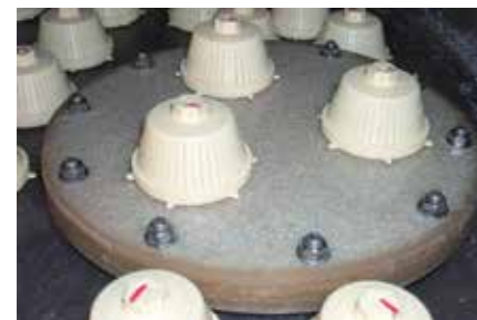
Internal Nozzle Plate Service Hatch
