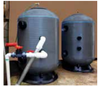
Using our 8-bar filter, the Wild Fisheries Program can now carry out tests to more than seven atmospheres.
